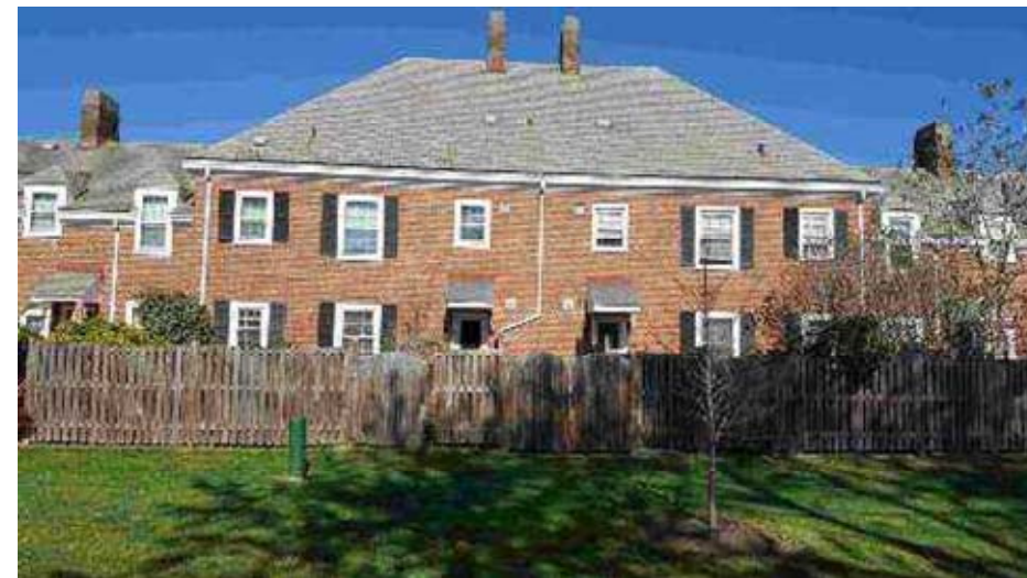
B UNITS – REAR PHOTO (2)
