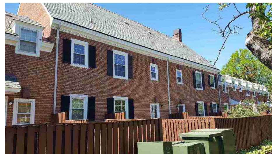
B UNITS – REAR PHOTO (1)
