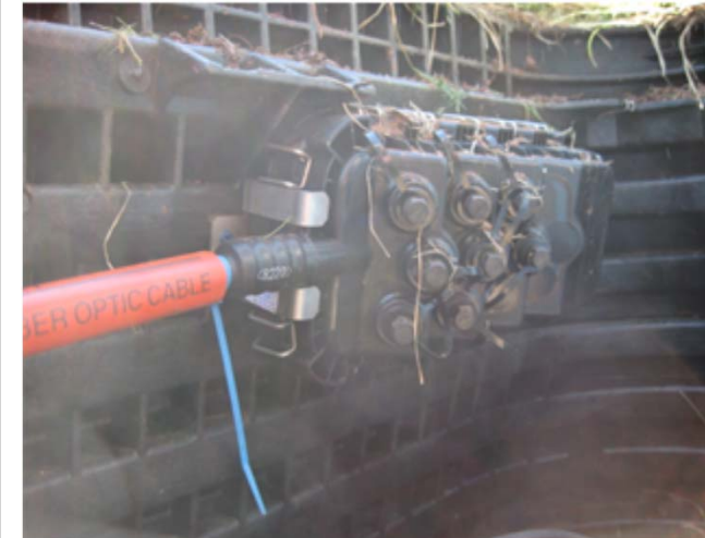
FB DT MOUNTED IN HAND HOLE (FOR ILLUSTRATION PURPOSES ONLY)
