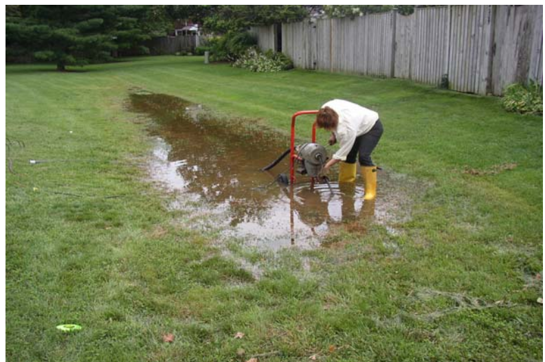
Glen Employee Maria Castro working on drainage behind Ct 11
