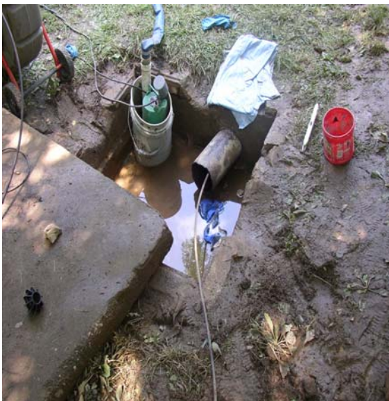
Original 1940's Storm Drain between Ct 2 and 3
