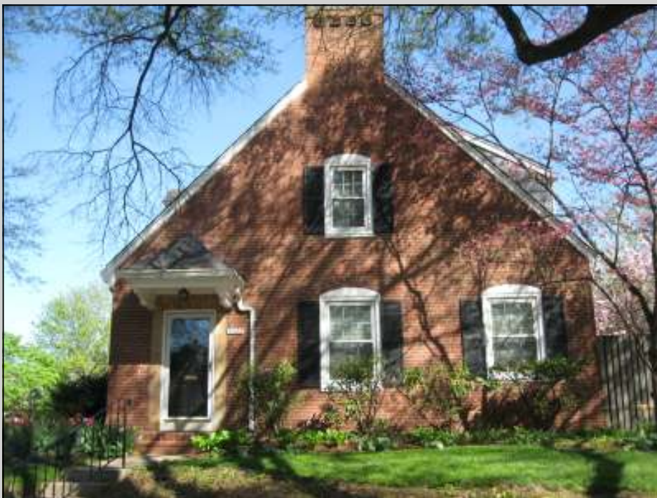
An example of a typical Fairlington Glen brick façade on this Edgewood unit.
