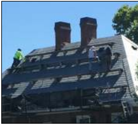
Workers replacing a Court 12 roof with new Vermont slate.
