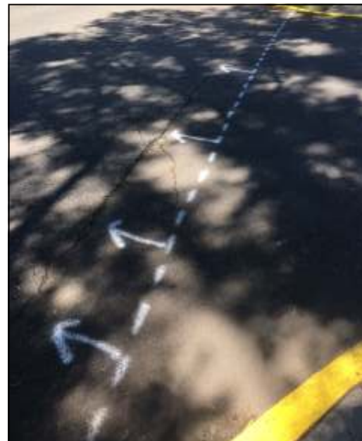
Markings like these will help County milling and paving crews know where the street ends and our parking lots begin.
