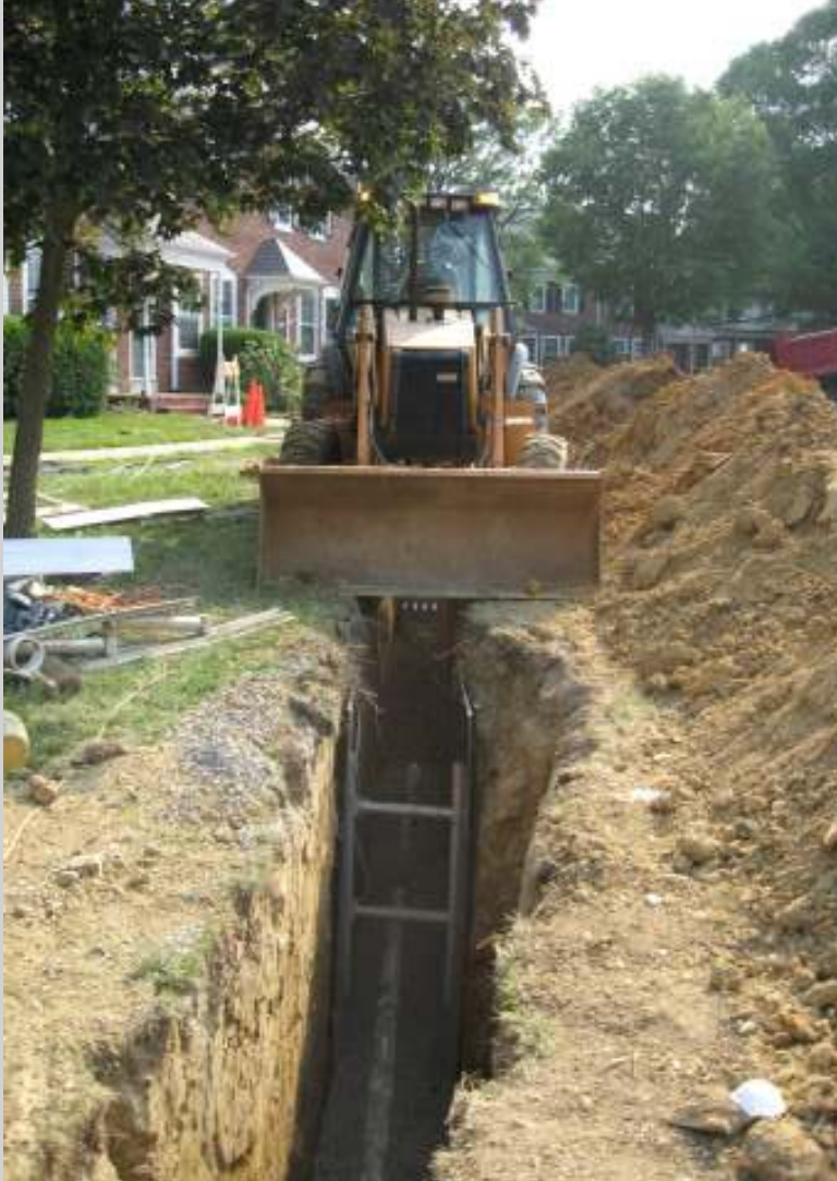
Construction workers dig a trench to reach one of the Glen’s sewer lines, which can be seen here below the surface of our common area grass.
