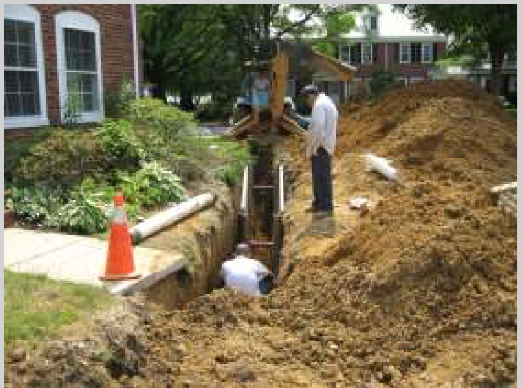
Construction crew works on a sewer lateral in the Glen.
