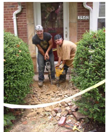
Court 12 Stoop Replacement.
