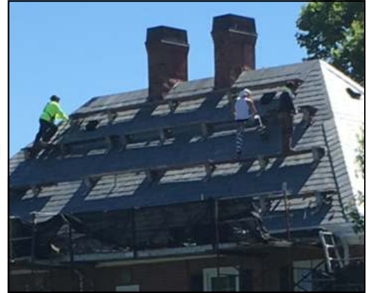
In 2017, roofers replace this Court 12 roof.
