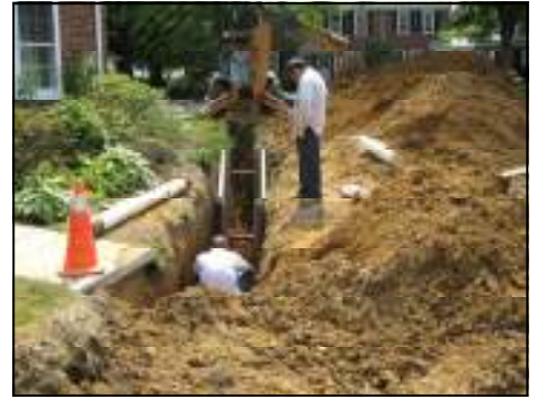
Work on a sewer lateral. (file photo)
