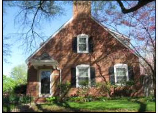
An example of a typical Glen brick façade on this Edgewood unit.
