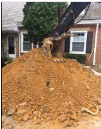
A partially collapsed sewer line was replaced in early September.
