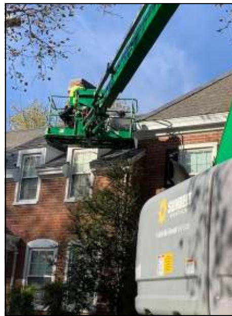
With the help of a lift, painters are able to reach the areas of buildings closest to the roofs.
