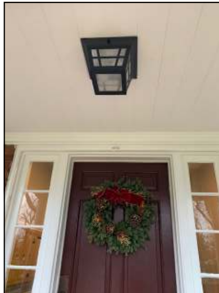
Even the front stoop lights were replaced with new fixtures and LED bulbs.
