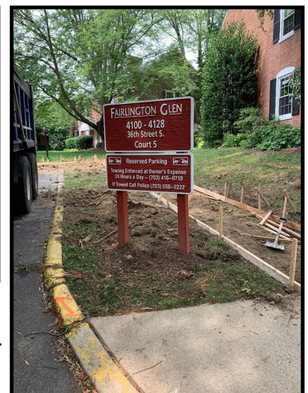
A new sidewalk will be installed just behind the Court 5 sign.
