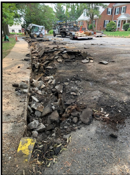
Work crews began the process of milling the existing Court 5 asphalt.
