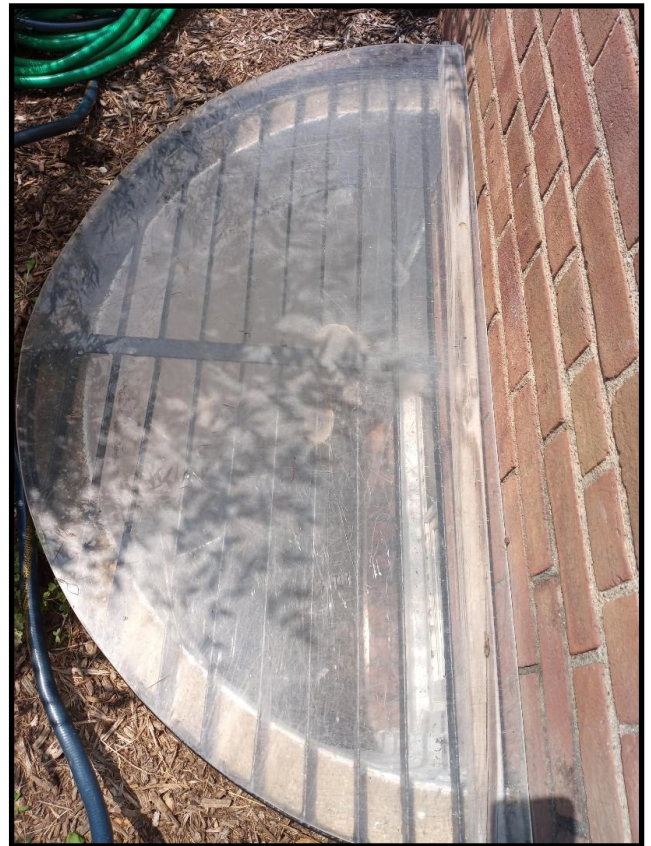
This flat Plexiglas window well cover is an example of what is approved in the Glen.
