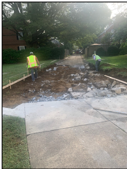
Dominion Paving crews beginning the same process in the Court 12/13 alley.
