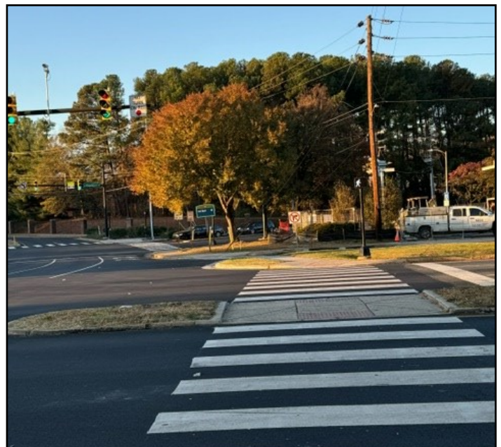
Mistake corrected! In this pic both the pedestrian walk signal and the green right turn arrow for cars is illuminated, causing a potential car/pedestrian accident.
