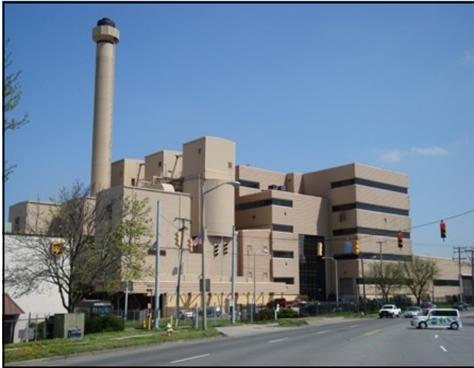
This Covanta Waste-to-Energy Facility on Eisenhower Avenue in Alexandria is where our trash is incinerated.
